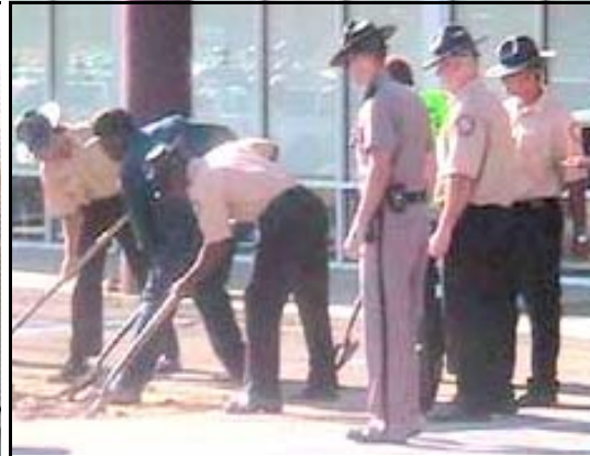
Troopers and C.W. Roberts Constructing, Inc., employees install speed bumps.
